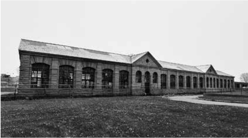
FIGURE 1.1 Adams Power Plant Transformer House today
