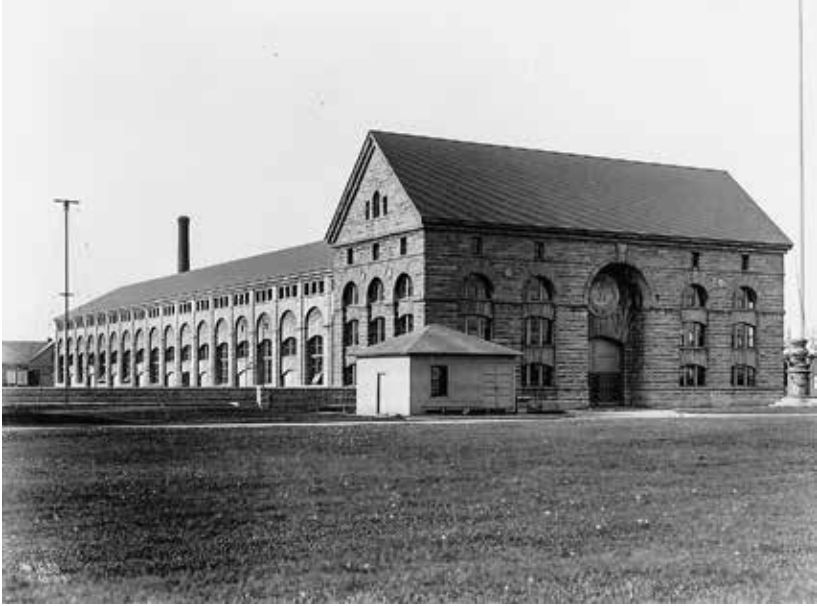
FIGURE 1.7 Adams Power Plant under construction. Niagara Falls Public Library, New York
