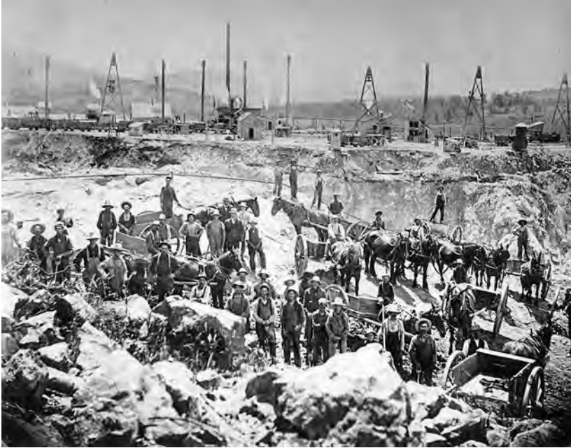
FIGURE 6 Stripping the land at the Jeffrey Mine, 1905
