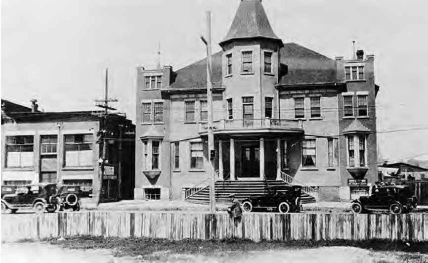
Finnish Labour Temple, Port Arthur, Ontario. 1920. Hoito Restaurant in basement. Työkansa Newspaper building on the left built in period 1912–14. (Photo courtesy of Thunder Bay Finnish Canadian Historical Society Collection, Lakehead University Archives.)
