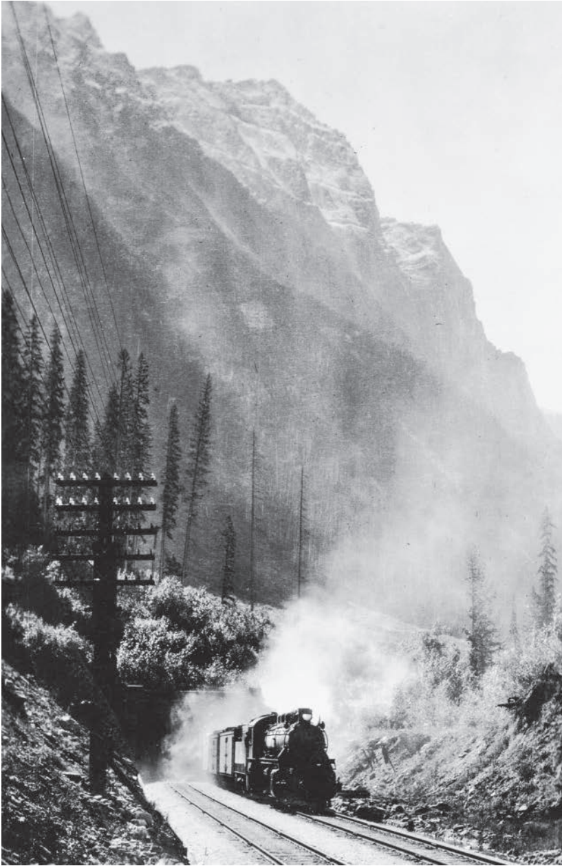
The east portal of the CPR's Connaught Tunnel at Mount Macdonald. Although it was a promise of Confederation, the last spike on the Canadian Pacific Railway was not driven until November 1885, fourteen years after British Columbia became part of Canada. | Courtesy Royal BC Museum and Archives, C-02516
