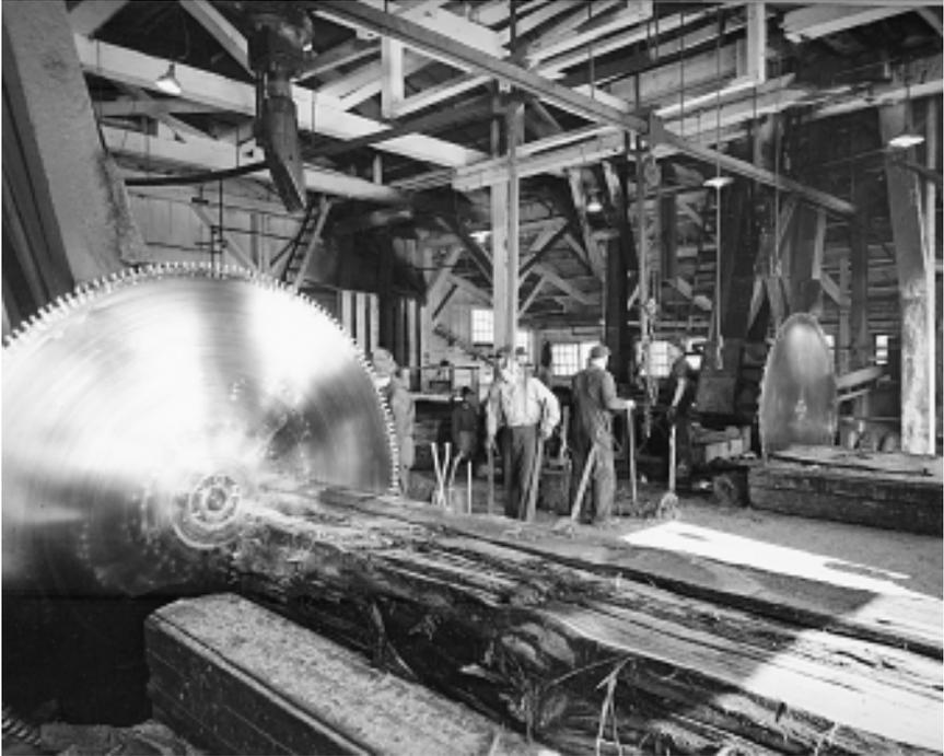
Cut-off saws in a Vancouver shingle mill, 1942.
