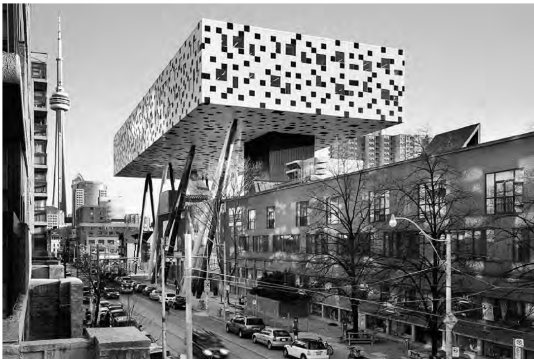
Figure 0.10 The Sharp Centre for Design, Ontario College of Art and Design, Toronto. | Photograph by Richard Johnson, www.interiorimages.ca .
